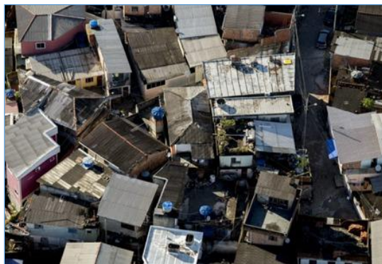
Figure 4. Aerial image of buildings in an irregular situation. DroneDeploy.
